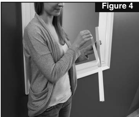
Step 4: Peel off double sided adhesive from behind the Miracle Channel.
