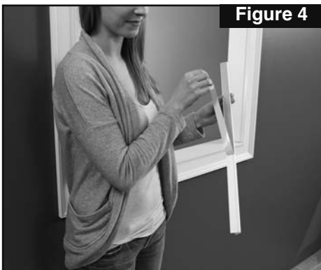
Step 4: Peel off double sided adhesive from behind the Miracle Fit Base.
